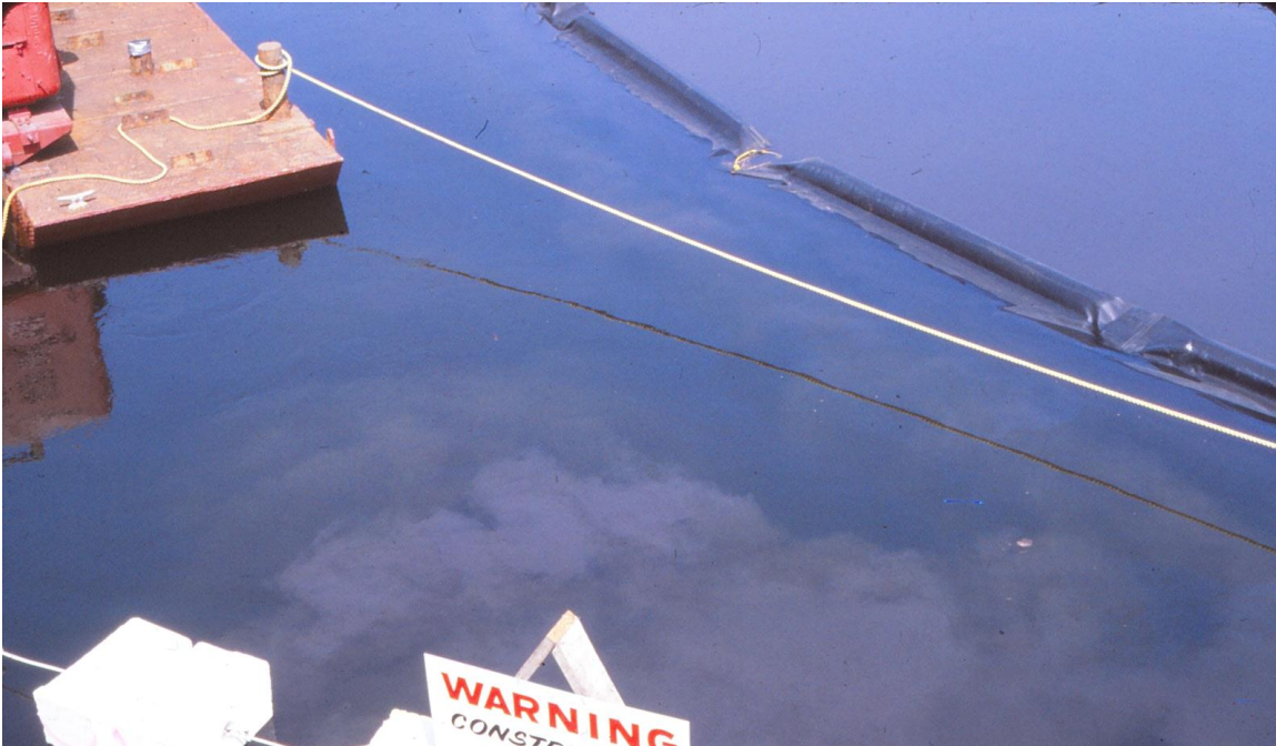
View of Exide's 1983 Lead remediation of Mill River sediments. The silt curtain to upper right is intended to separate the resuspended sediment within the active dredge cell from the protected open water in the river located to the left. Note the boiling clouds of resuspended sediment blowing out from beneath the curtain into the open river water between the rope and the warning sign. April 1983 tjs
