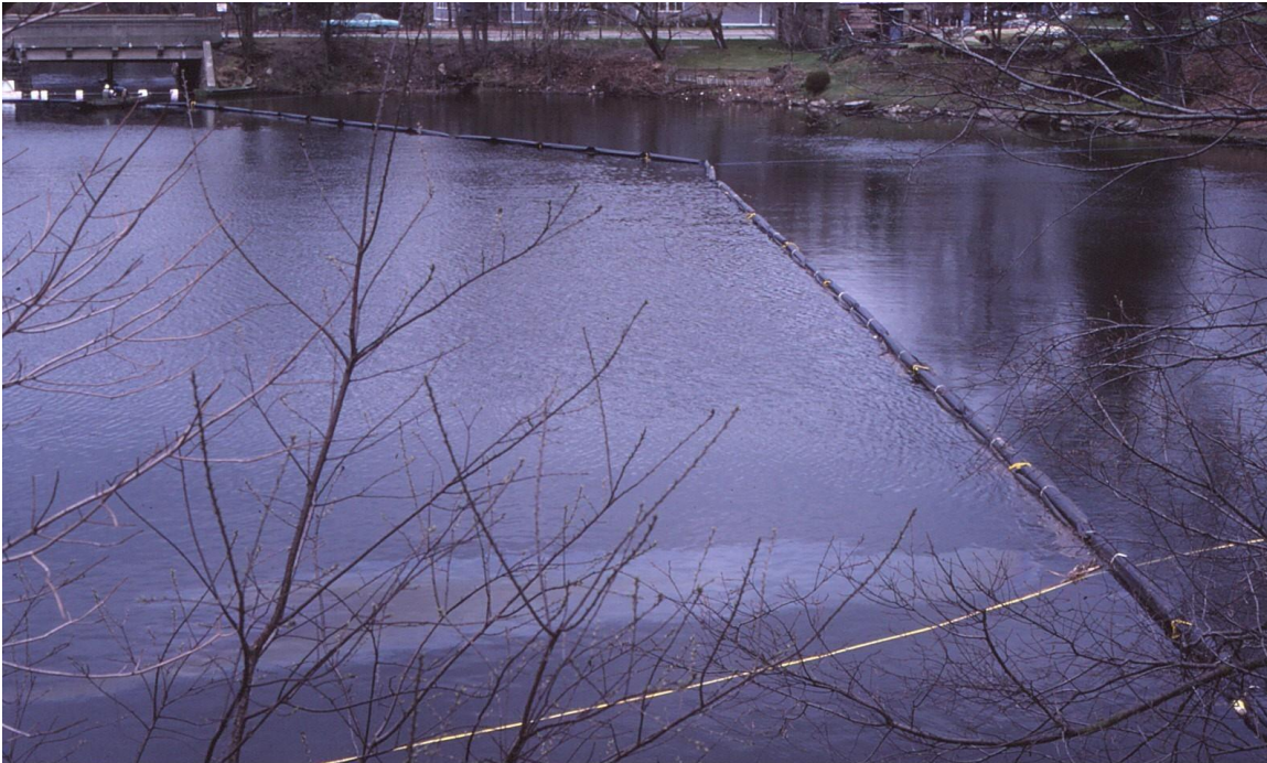
View of Exide's 1983 remediation of Mill River mill pond looking from the railroad toward the Post Rd. The dredge cell silt curtain to the right is suspended from the floating boom and is intended to protect the open water in the Mill River. Note the oil slick in the foreground contained within the boom. April 1983 tjs
