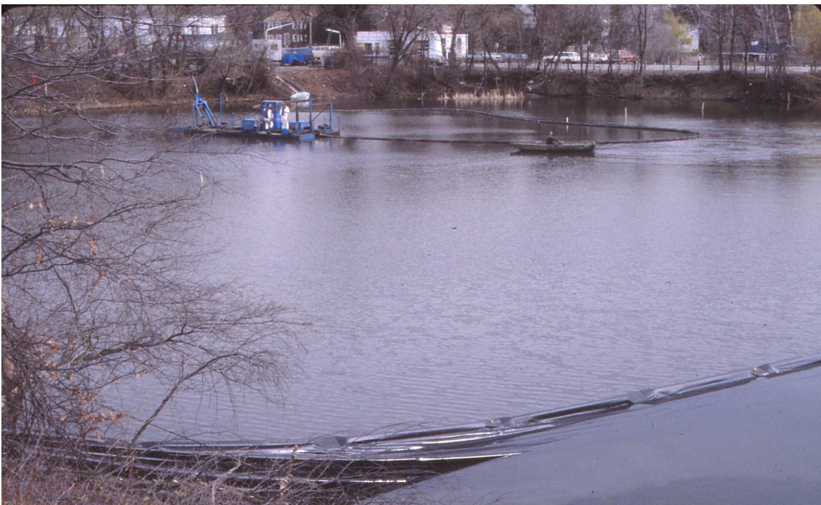
View of Exide's 1983 Mill River Lead remediation project. Note silt curtain suspended from floating boom with resuspended sediment discharging from under the curtain in the foreground. Depending on the tide, river flow, rainfall, and dredge pumping, the resuspended sediment discharged over, around, and under the silt curtain into the open river. April 1983 tjs
