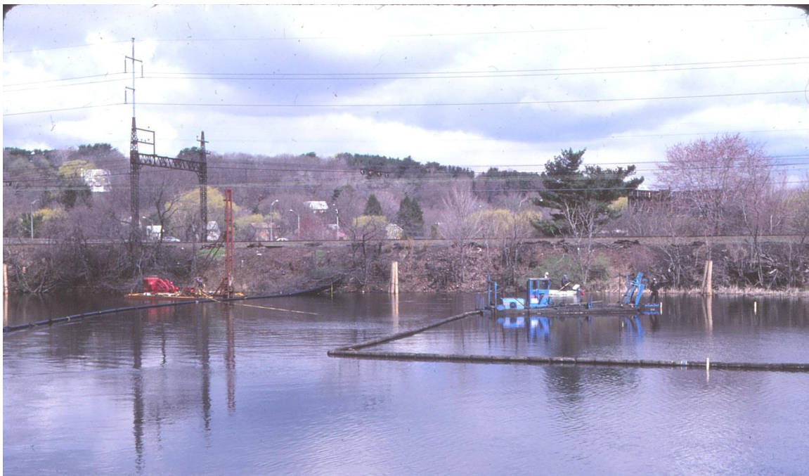
Looking northerly at Exide's 1983 Lead remediation project in Mill River sediments. The floating silt curtain is deployed around the dredge cell on the left side to protect the open water in the river; the pile-driver is installing timber support piles for shifting the dredge on cables; the hydraulic cutterhead dredge is dredging the bottom sediment and pumping it through a floating pipeline to the treatment and disposal area. April 1983 tjs
