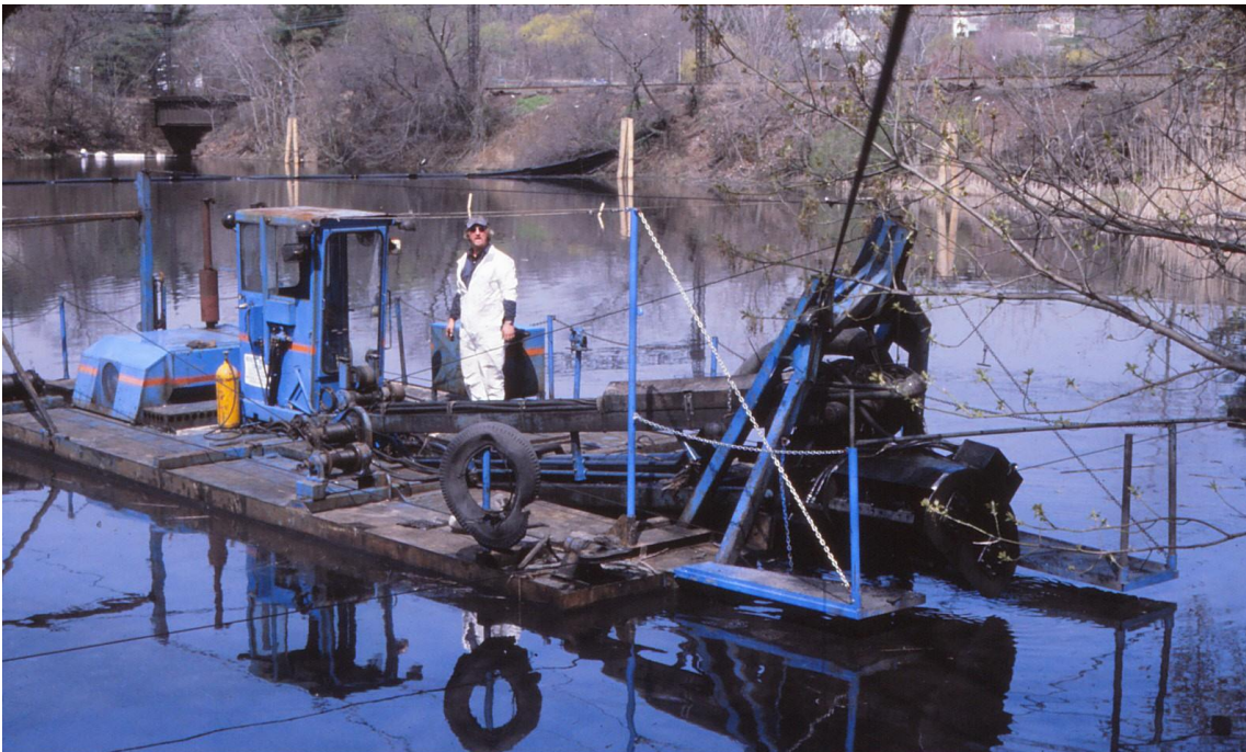
View of the 1983 Exide Mill River sediment remediation project. This is a hydraulic cutterhead dredge with shroud, variable-speed pump and cutterhead. The dredge shifts its position by moving along a cable suspended between timber pilings located around the shoreline. April 1983 tjs
