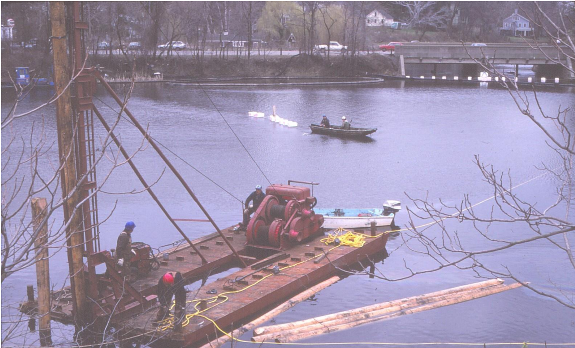
View of Exide's 1983 Mill River sediment Lead remediation project. The work barge in the foreground is driving timber piling along the shoreline to support the cable for shifting the dredge as it cuts into the river bottom.'83 tjs
